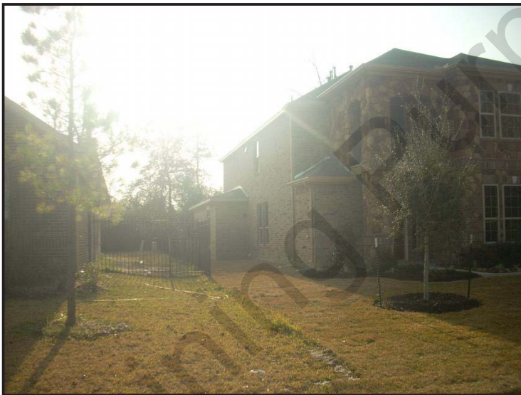
Side of Subject Property
