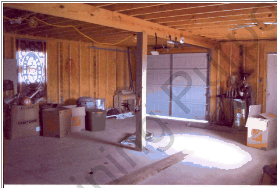
INTERIOR OF DETACHED GARAGE/ SHOP
