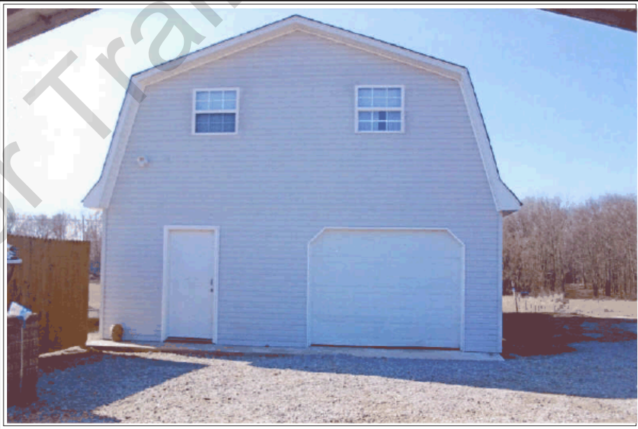
DET GARAGE/SHOP WITH FINISH BONUS/ BATH
